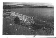
Collapsed gabions have left the soil completely unprotected from the force of the sea. They are also not very attractive.
