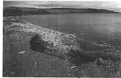
Collapsed gabions have left the soil completely unprotected from the force of the sea. They are also not very attractive.
