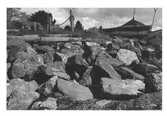
If you present a slope of large rocks which interlock; the force of the waves crashing against them will push the rocks downwards and therefore secure the rock slope. A disadvantage to this method is that because it is a slope; on a particularly stormy day, waves will crash over the rocks onto land.
