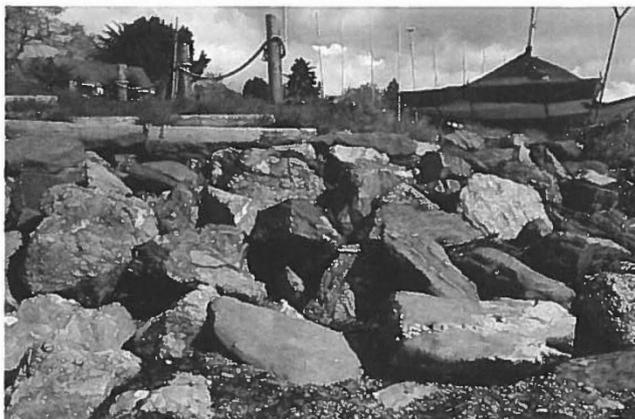
If you present a slope of large rocks which interlock; the force of the waves crashing against them will push the rocks downwards and therefore secure the rock slope. A disadvantage to this method is that because it is a slope; on a particularly stormy day, waves will crash over the rocks onto land.
