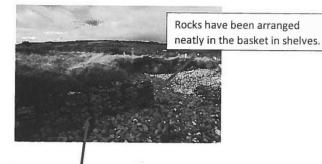
Gabions are at a slight angle to reduce the force of impact from the waves.
