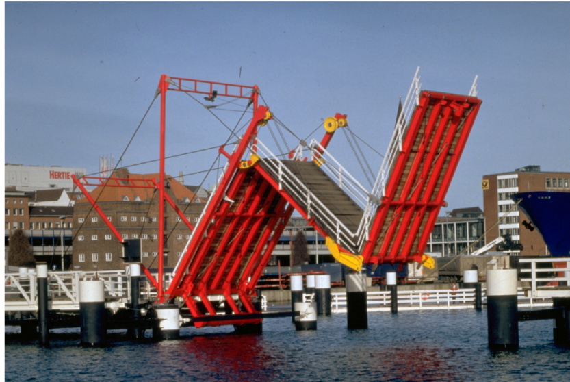
Figure 1: Hörn bridge during the folding process (schlaich bergemann partner, no date)
